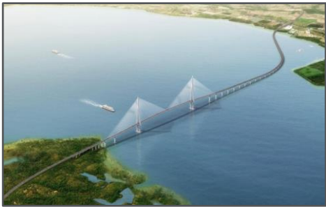
Panay-Guimaras-Negros Inter-Island Link Bridge – PHP187.5bn (US$3.3bn)
