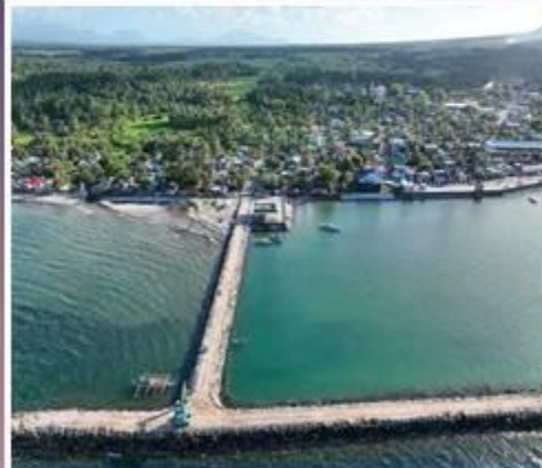
Bacon Blvd Breakwater Structure, Sorsogon City
